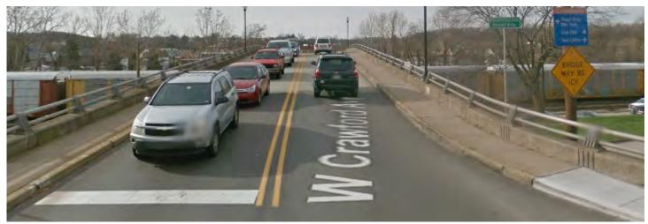
Safety problems currently represent barriers to bicycle and pedestrian mobility within Connellsville. The Crawford Bridge crossing shown here is one example, combining heavy vehicle volume, slope, narrow sidewalks and low safety railings.
