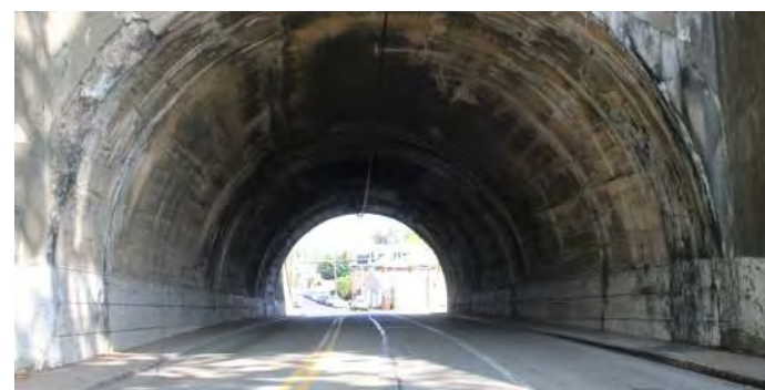
Arch Avenue Tunnel
