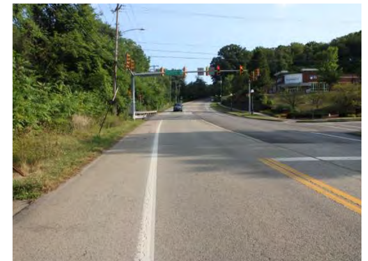
N Main Street Corridor
